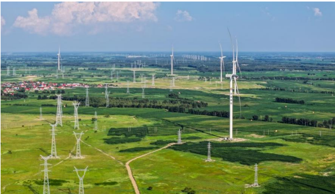
Figure 3, Inner Mongolia Tongliao 2.38 Million Kilowatt Wind Power Project (Source: Xinhua News)
